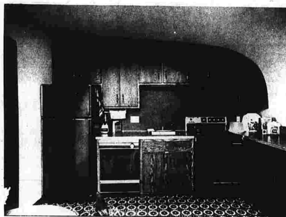
Contour of kitchen cabinets conforms to shape of panels.
